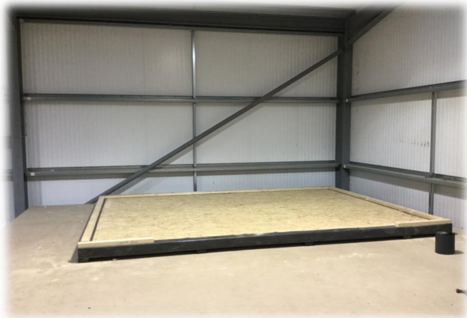
Image above showing a floor complete with floor plate arrangement.
